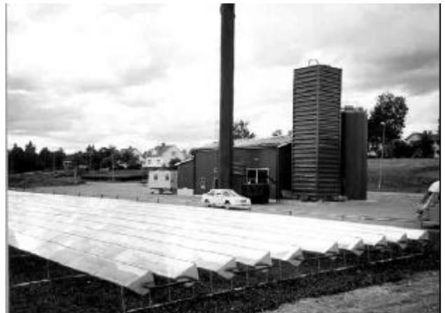
**Fig. 13** Pilot plant with 500 m<sup>2</sup> MaReCo collectors in Torsåker 1999. Photo: VUAB.
