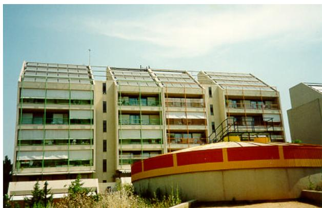
**Fig. 17** Lykovrissi with seasonal storage tank in front of the heated building.
