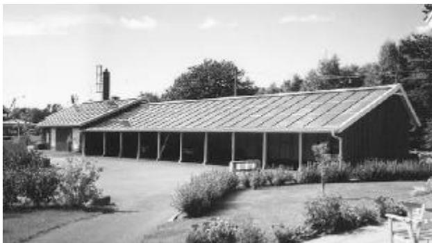
**Fig. 14** 220 m<sup>2</sup> roof module collectors in Onsala. Photo: Jochen Dahm
